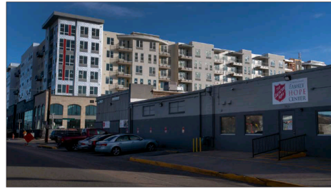
ABOVE: The Weidner Apartment Homes, an upscale complex under construction, towers over the Salvation Army's Montgomery Family Hope Center on South Sierra Madre Street. When residents of the Mill Street neighborhood express concern over gentrification of the area, they often refer to the stark contrast between the new high-rise apartments and the Salvation Army's shelter.
